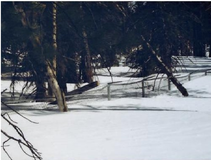
Snow buries 6 foot fence around tank. Fallen trees demolish portions of fence.
